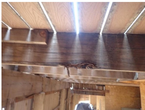
Figure 2 – Damaged Joist
