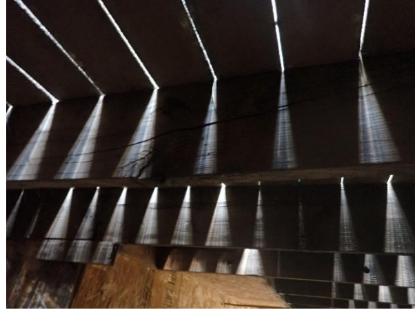
Figure 5 – Split Joist
