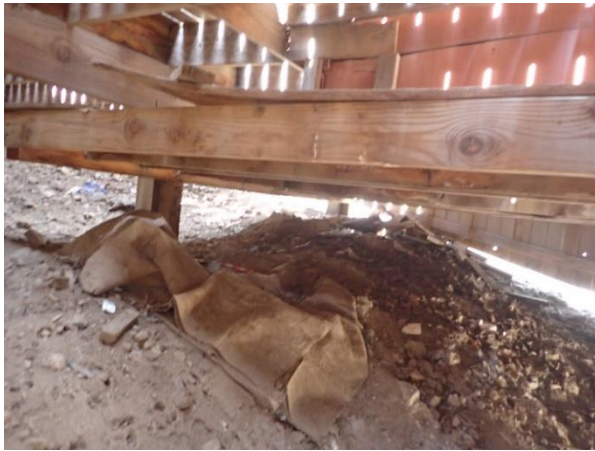
Figure 1 – Typical Original Framing
