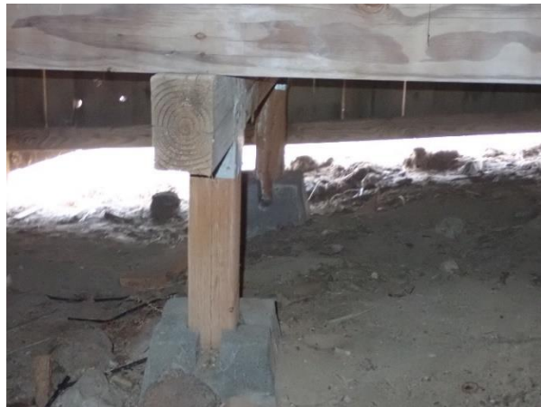
Figure 5 – Typical Renovation Post
