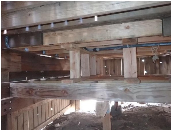
Figure 4 – Typical Unbraced Renovation Framing
